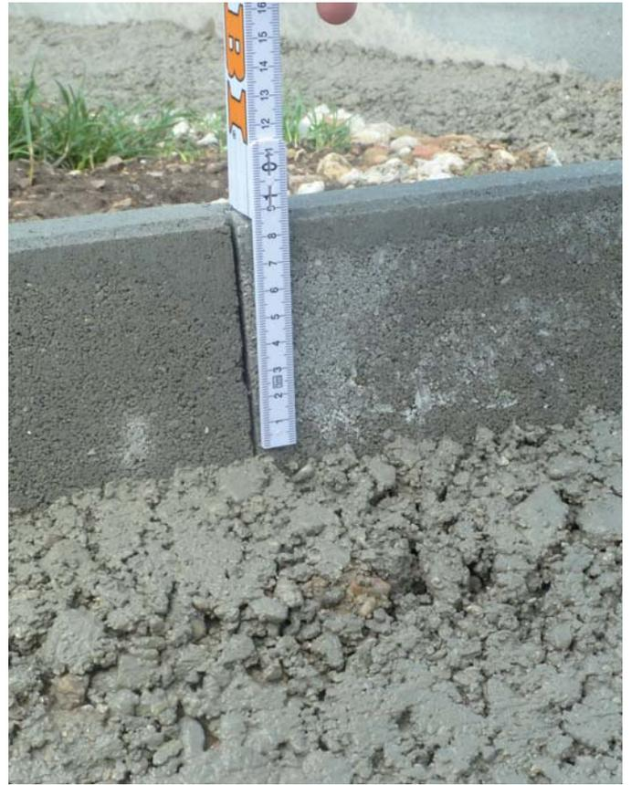
Abb. Betonrandsteine OK Fundament = < -8cm 20.5.2016; 10:46
